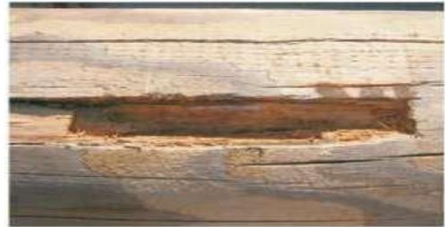
*Cleaned out decayed pocket with some loose wood fibers.*
