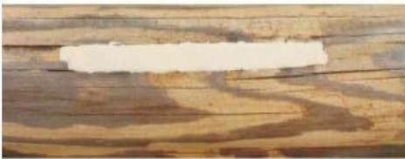
*Cavity filled with E-Wood.*
