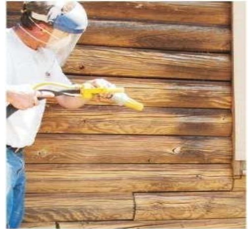
Media blasting with crushed glass
