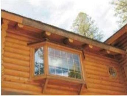
Section of fascia that was wire brushed.
