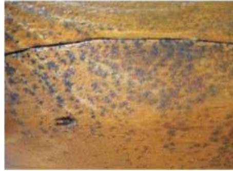
Iron tannate discolorations from an unknown source.
