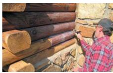
The application of *Prelude*<sup>TM</sup> is much the same as the finish application; use an airless and spray until the point of run-off and back brush to work it into the fissures and checks on the logs as well as to brush out any runs. You can also use the "brush and bucket" method if you're one of the traditionalist types. It dries fairly quickly and cleans up with soap and water.
